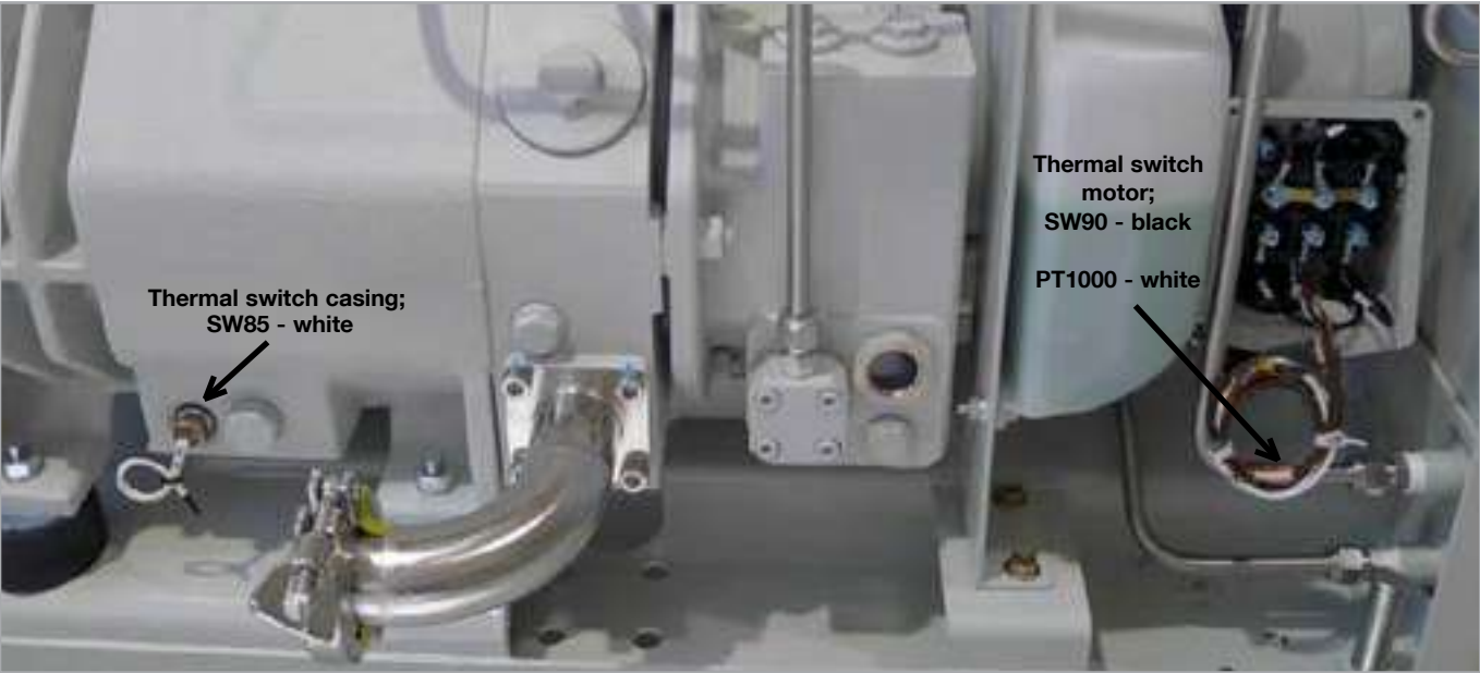
Fig. 3.3 Thermal switch positions
